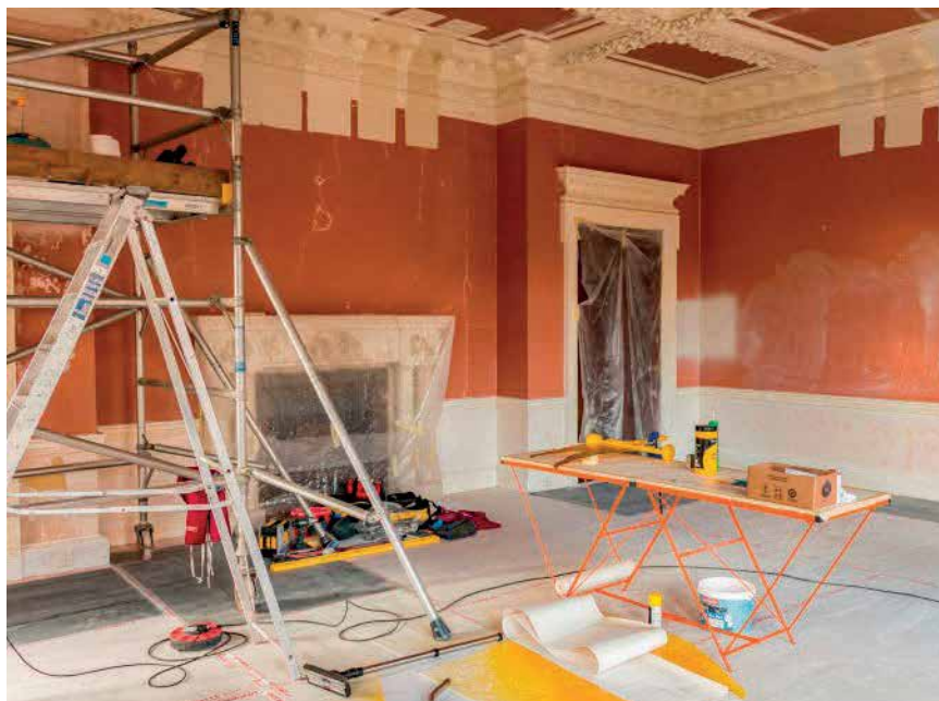
The Music Room in the West Wing undergoing conservation work.
